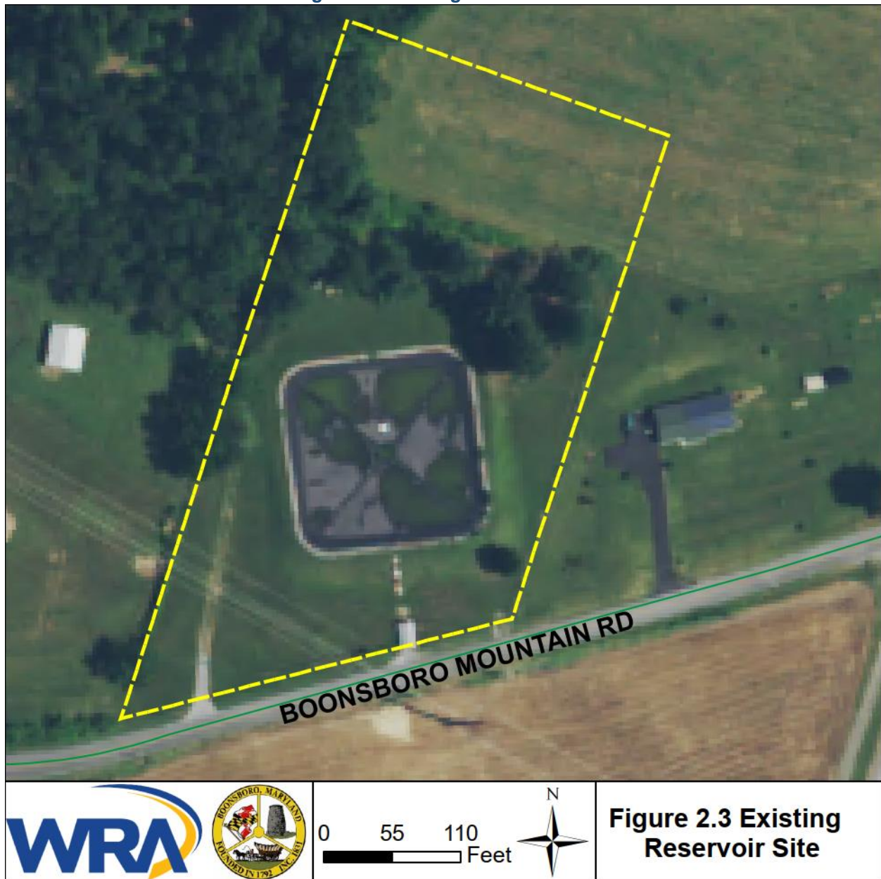
Figure 2.3 Existing Reservoir Site
