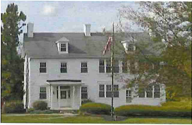
EXISTING FARMHOUSE BUILT IN OR AROUND 1880 -1890
